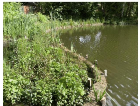
Reed and coir rolls placed in Little Dawley Pools to create a natural green barrier
