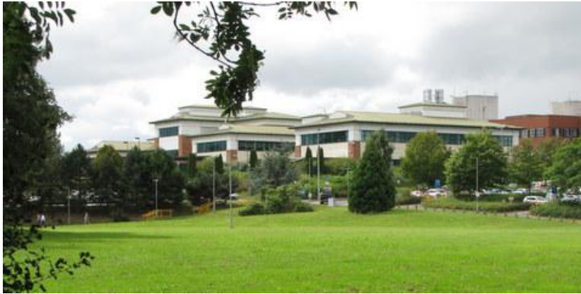
The main building and Post-Graduate Medical Centre at County Hospital, Stafford
