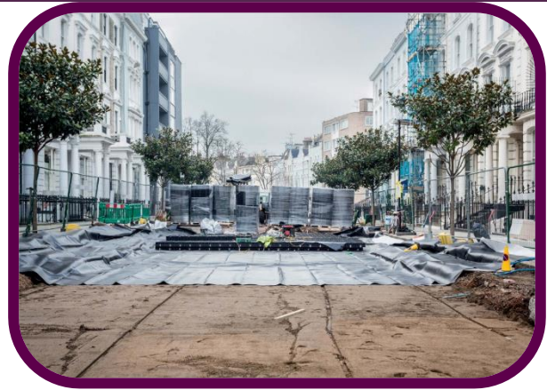
Image: The SuDS scheme being constructed © SEL Environmental
