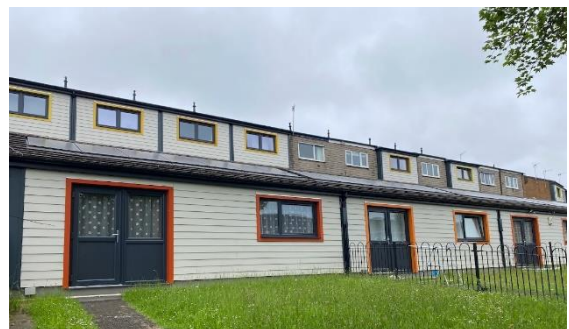
Whole-house retrofit work © Nottingham City Council
