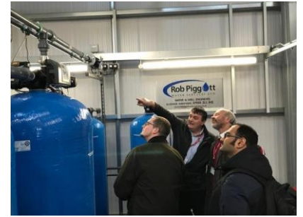
The STEP Energy Centre
